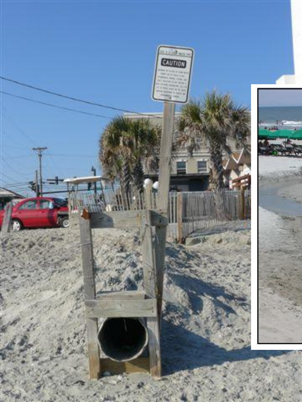
Stormwater Pipes on the Beach Face
